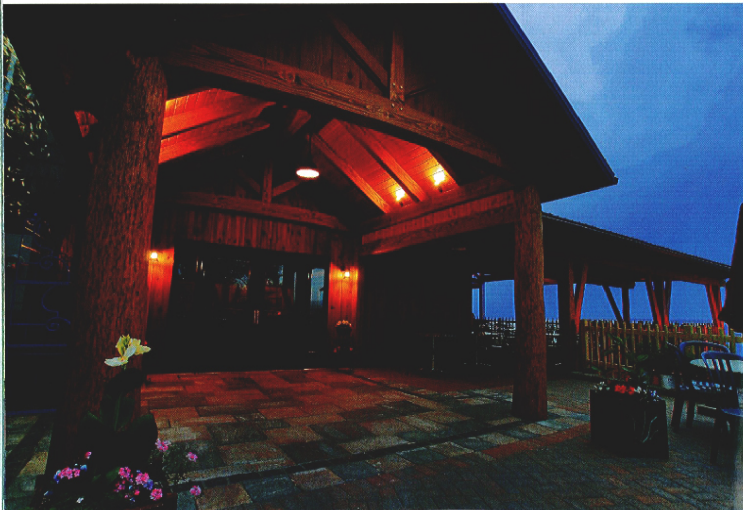
Peeled beams and an expansive timber frame immediately convey craft and quality, reflecting the food and wine at Bully Hill.
